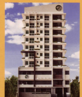
Baron 3 Gardens (Completed)
