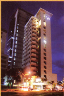
W Tower (Completed)
